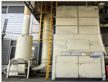
[Filter dust collectors in the R&D Center]
