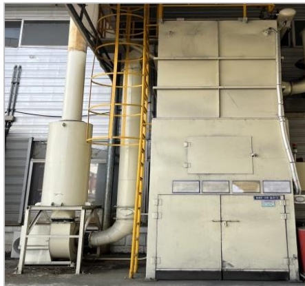
[Technology Research Center Filter Dust Collector]
