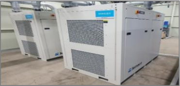
[Highly efficient air dryers]
