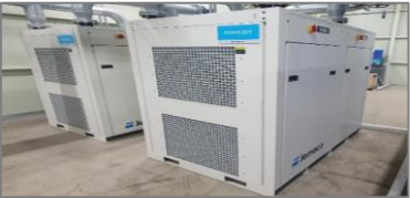
[Highly efficient air dryers]
